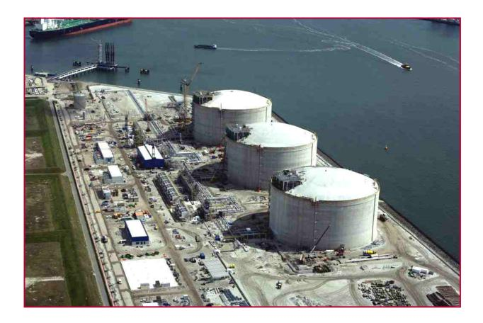
Steels which have been used under ambient temperature are usually called low temperature service steel. Main applications are storage and transportation vessel for liquefied gases. To maintain gases at the liquefied state, the easy way is to decrease temperature. It is understandable that storage vessel as well as the other auxiliary machinery should be ready for low temperature service.
